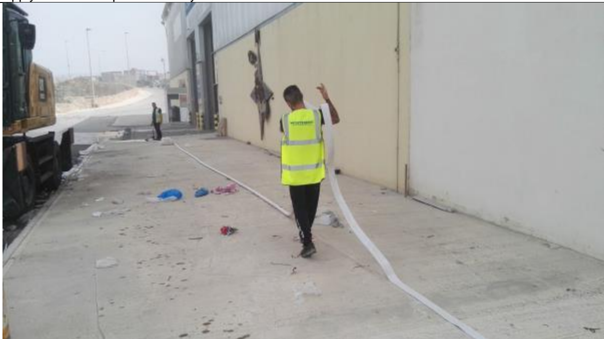
STEP 6: Drain all the water from the fire hose.
