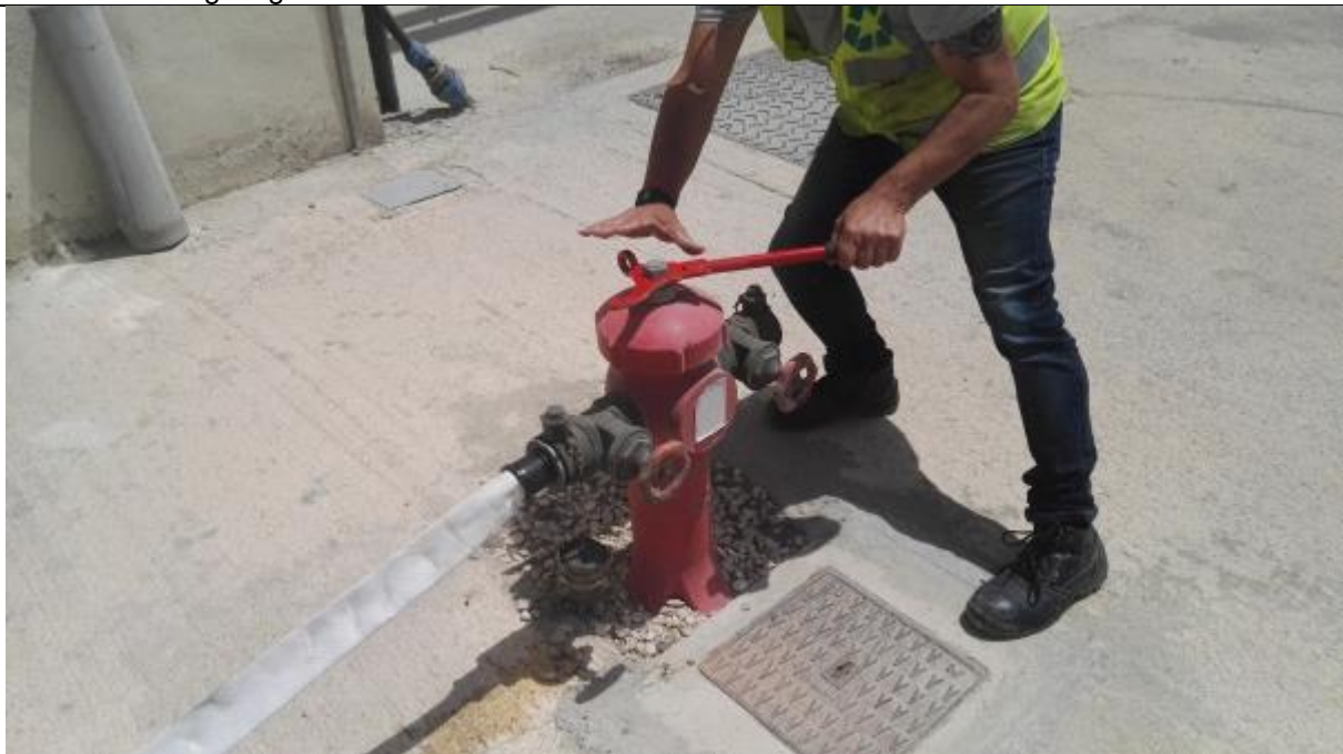
STEP 4: Unscrew the nut at the top of the fire hydrant using the fire key.
