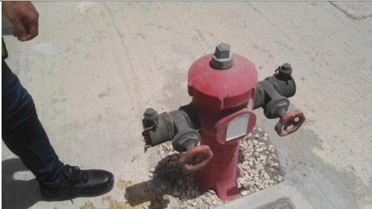
STEP 5: Apply the outlet cap to the fire hydrant.
